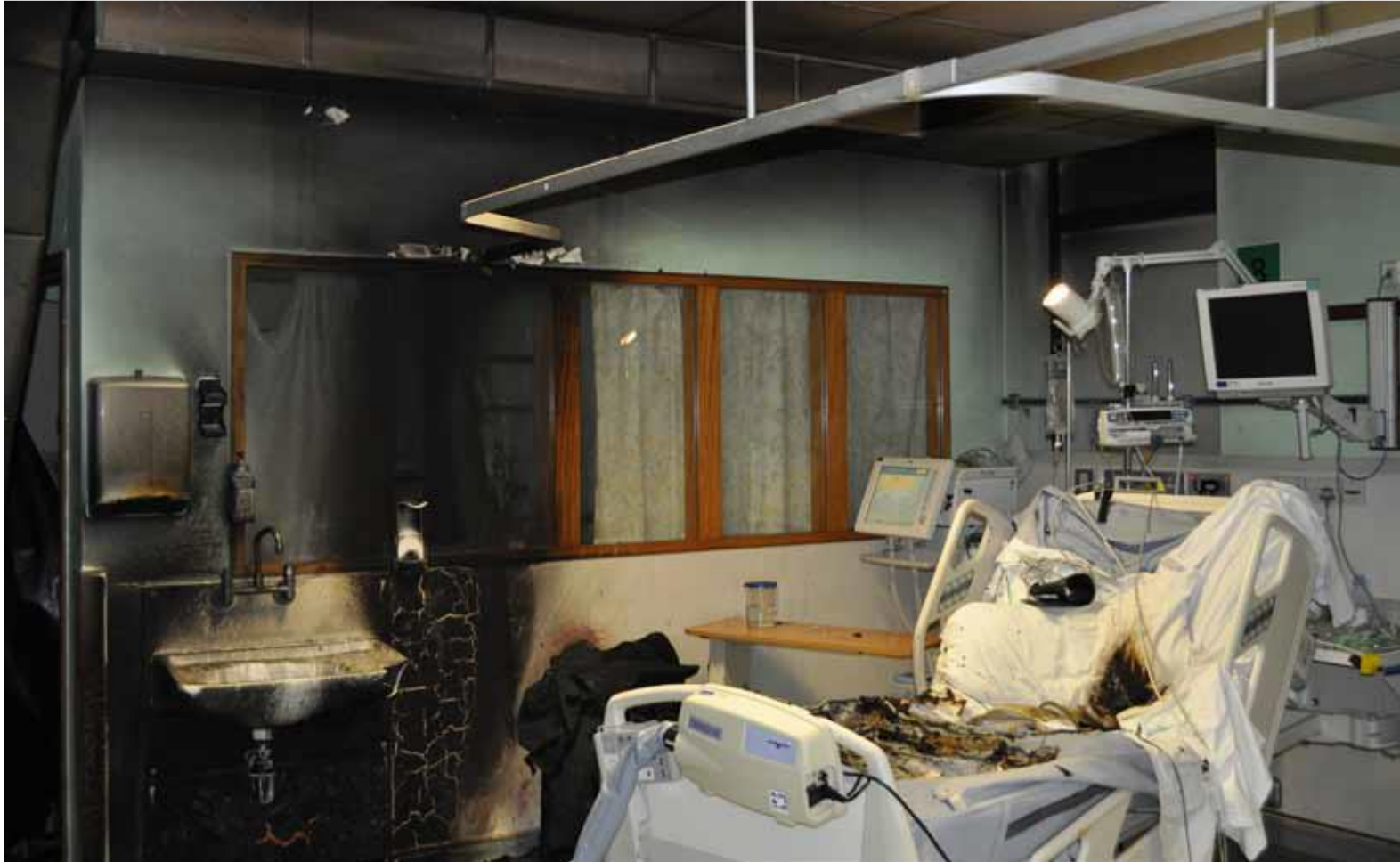
Flona Kelly, "Fire on intensive care caused by an oxygen cylinder", Anesthesia News, 2013
